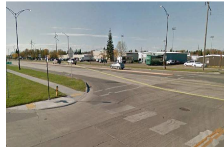
Existing Pedestrian Ramps
